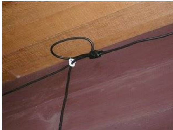
Photo 32-4 Extension cords used at permanent lighting in living room.
