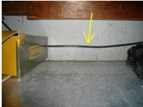
Photo 32-2 Unsupported wiring in garage workbench cabinets.
