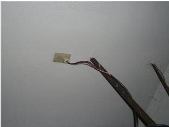
Photo 32-1 Extension cord used at garage door opener w/ unprotected wires.
