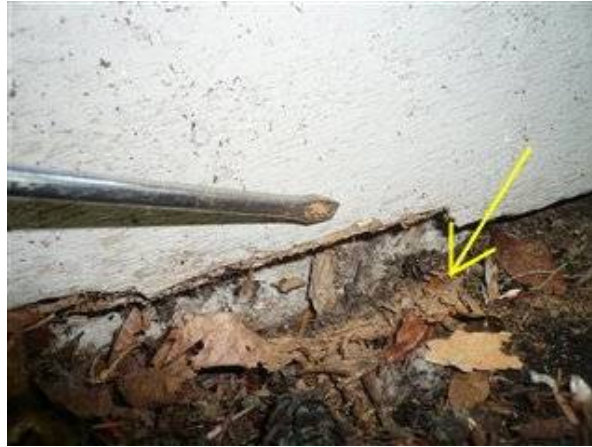
Photo 66-2 Siding damaged by anobiid beetles with frass below.
