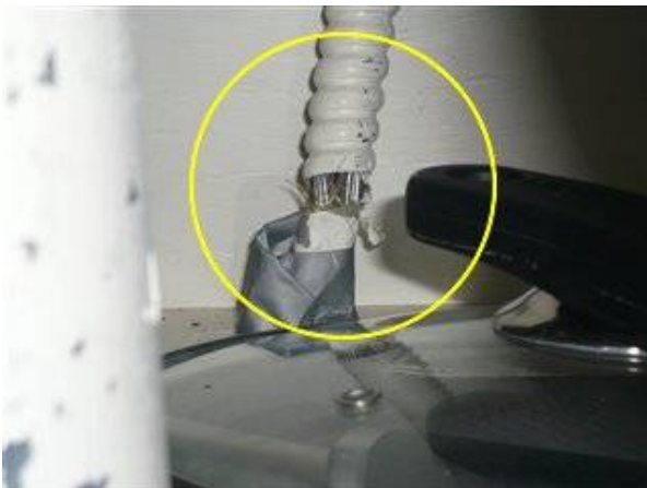
Photo 32-3 Damaged shielding/exposed wires in cabinet below cooktop.
