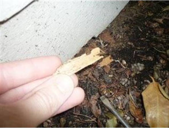
Photo 66-1 Anobiid beetle galleries in damaged siding.
